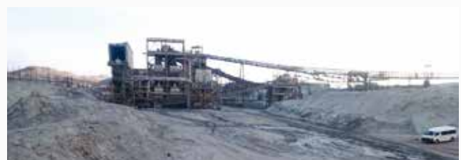
Progressive rehabilitation under way — (above) before rehabilitation; (below) after rehabilitation.
