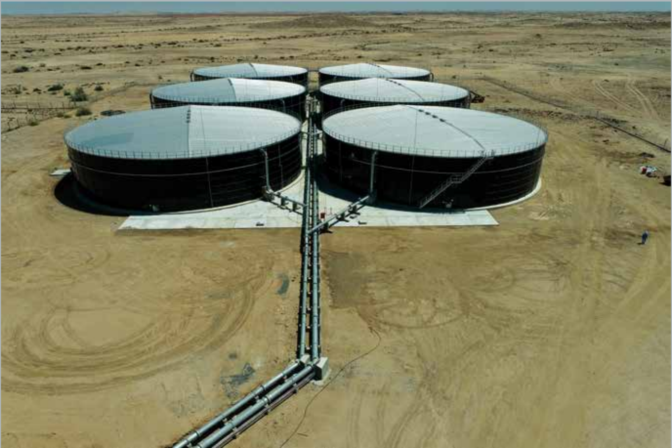
The six water storage tanks were completed in 2021 and will increase the mine's water storage capacity with 60,000 m 3 .
